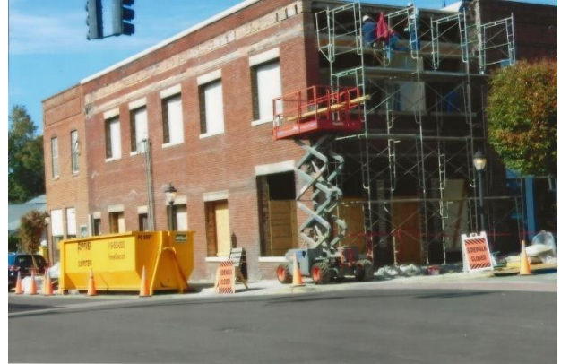
Former Farmers & Merchants Bank now being restored
